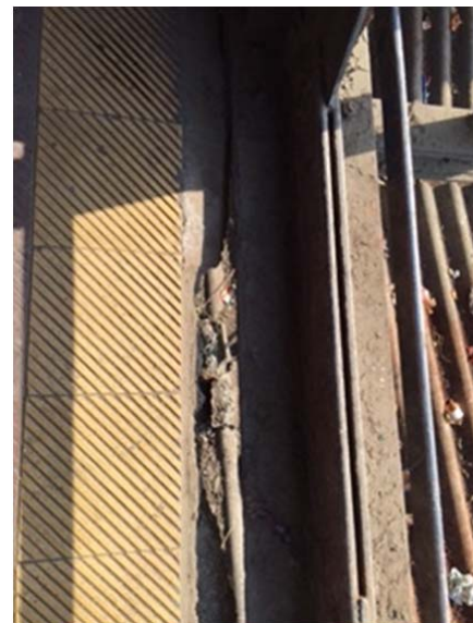
Figure 9: Gaps on the corners of FOBs
